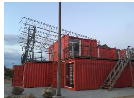
The E&P House - In Gellerup the E&P House is a place everybody knows. But for those who do not just live in the area, here is a photo. And 'yes' - the 'house' is a number of containers stacked on top of each other.
